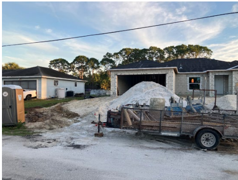
Figure 1- Swale is being blocked from a pile of dirt and porta potty, also is missing temporary culvert pipe.
