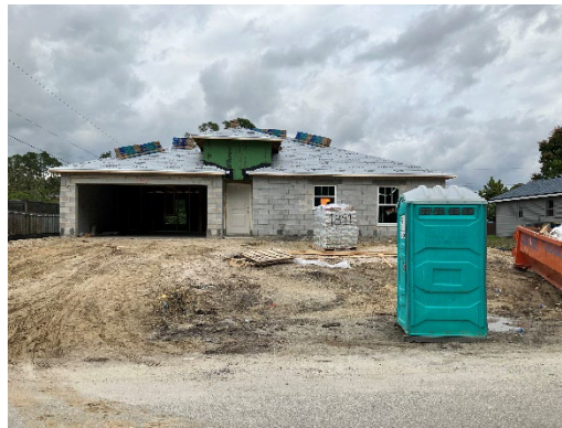
Figure 3 - No temporary culvert installed, porta potty and dumpster in the swale.
