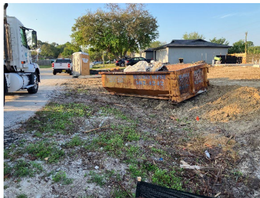
Figure 2 - Swale is being blocked by dumpster and missing temporary culvert pipe.
