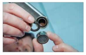
Clean Aerators-Aerators are small attachments at the tips of faucets which regulate the flow of water. They can accumulate small particles of lead in their screens. It's a good idea to remove your aerators at least monthly and clean them out.
